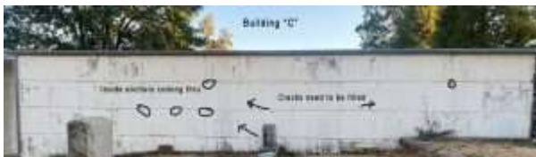
Prior to Repair and Painting
